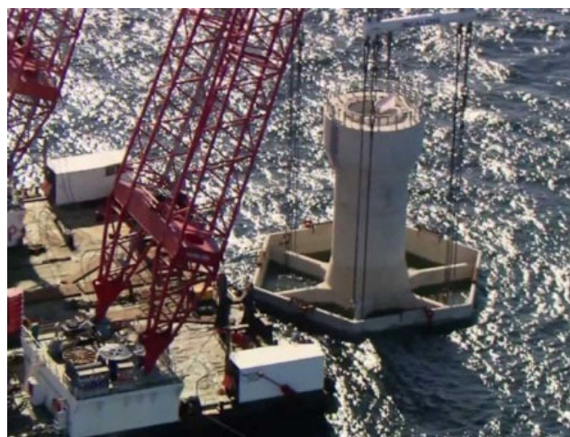
Fig. 5. Installation of the supports (Ruiz de Temino Alonso, 2013)
