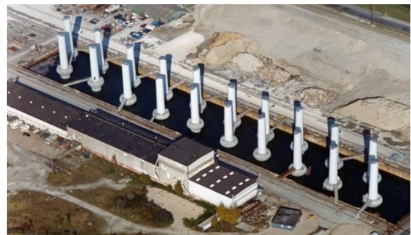
Fig. 2. Construction of supports in dry dock (Ruiz de Temino Alonso, 2013)
