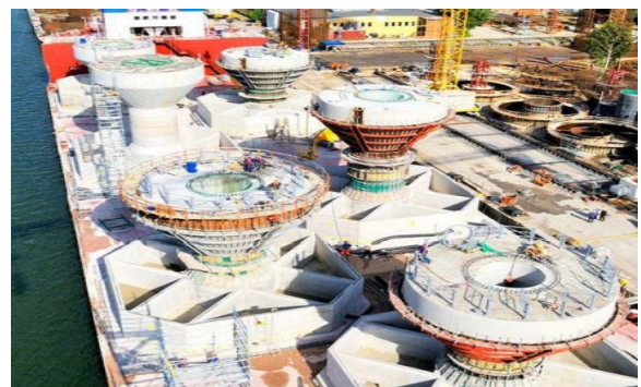
Fig. 3. Construction of supports on semisubmersible barge (Ruiz de Temino Alonso, 2013)
