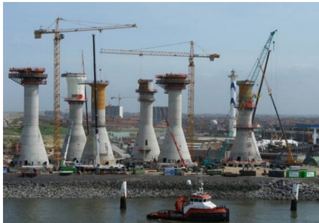
Fig. 4. Construction of supports on the quayside (Ruiz de Temino Alonso, 2013)
